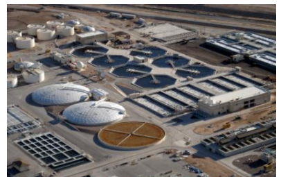
Aerial view of a typical wastewater treatment plant
